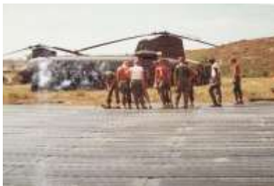
Laying PSP in Maintenance area
